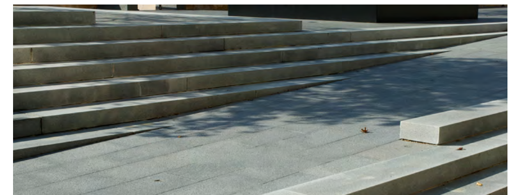
Stair / Ramp at Hotel Lobby
