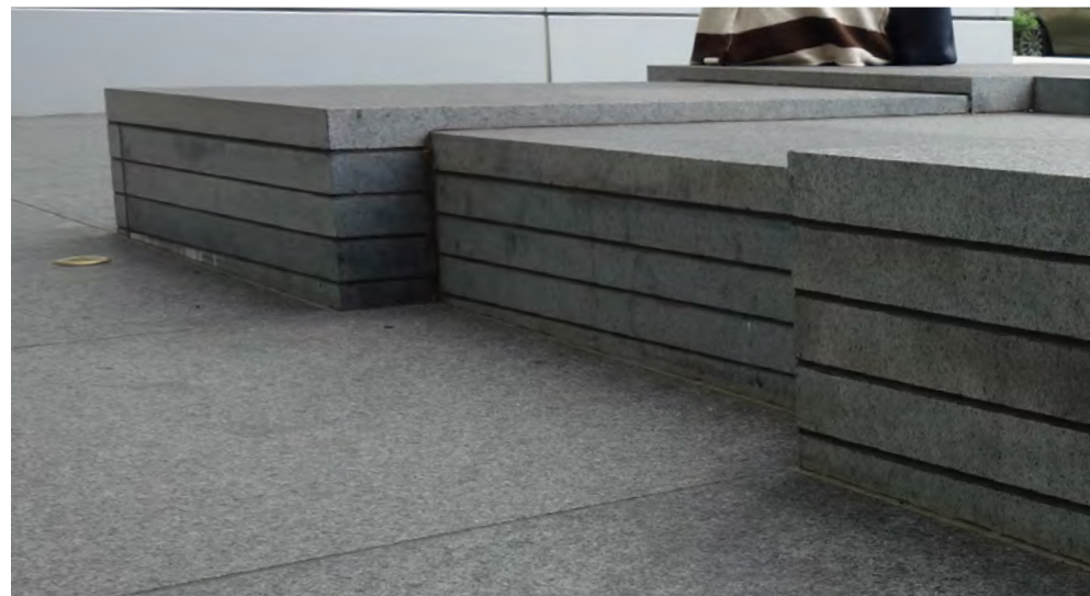
Granite Retaining Wall
