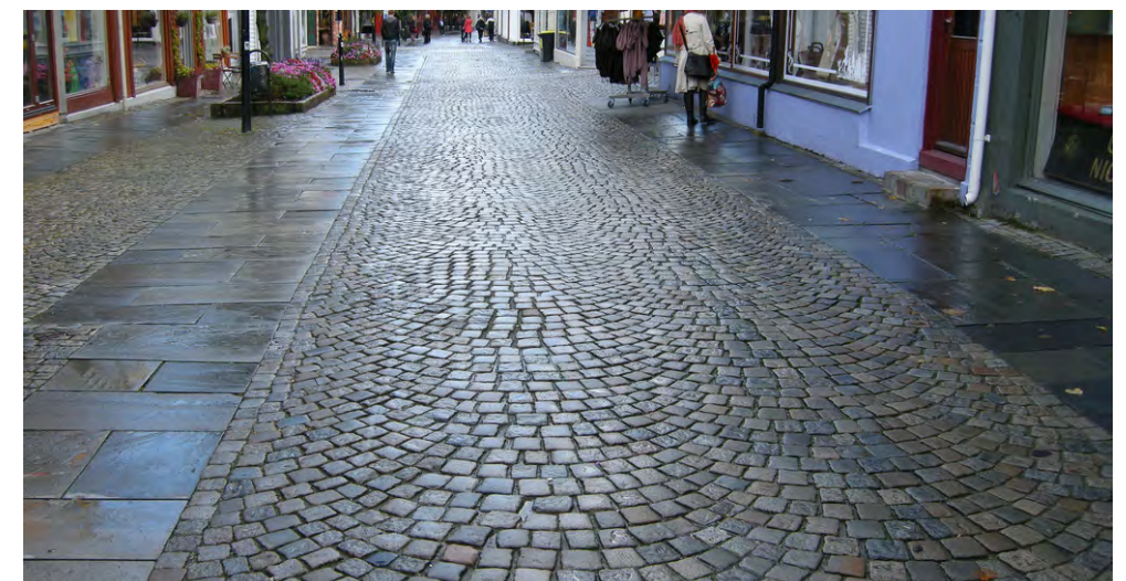
Curbless Paving and Vehicular Overlapping Paving
